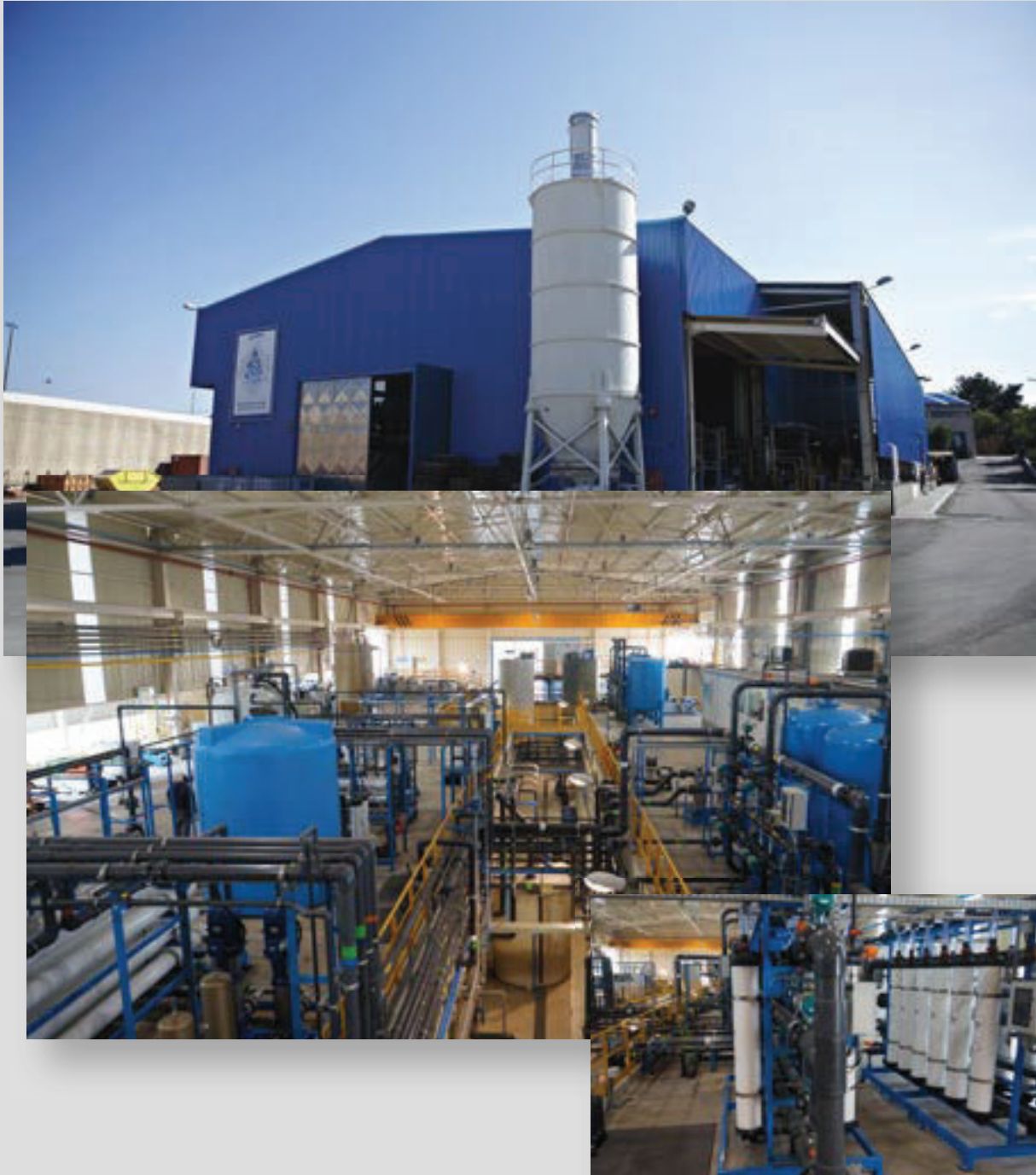
Industrial Water Treatment and Recycling Facility
